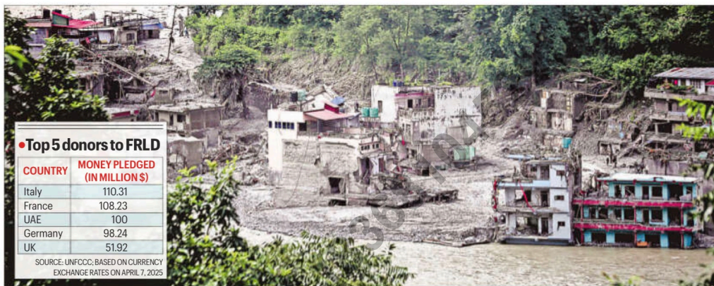
The devastated structure around Betrawati Rasuwa border in Nepal following the flash floods on August 31. FILE
