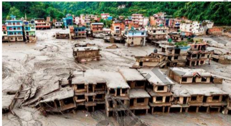
Swept away: Sludge surrounds damaged buildings at Bidur in Nuwakot district of Nepal on Thursday, more than 24 hours after the deadly flood tore through the region. AFP
