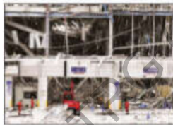
Rescuers work at the damaged Aeon Mall in Japan's Kumamoto prefecture on Wednesday. AP
