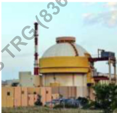
The reported data leak comes amid construction of four VVER reactors at the plant. FILE PHOTO
