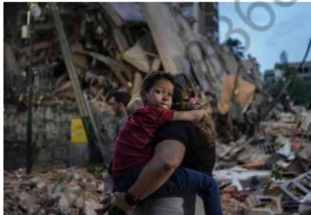
Lost in seconds: A woman holds a boy near a collapsed building in Caracas, Venezuela, on Thursday following the earthquakes. AFP
